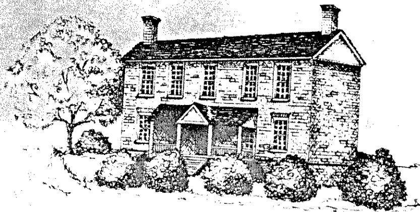
Built in 1813 by Charles Scott, Melrose was home to the Shores, Tutwiler, Johnson and Seay families. Greek Revival pediments, a refined water table and corner "rubbed bricks" are gracious touches which offset the unusually tall proportions.
